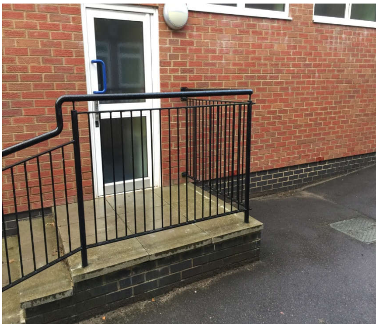
Build ramp from right.
